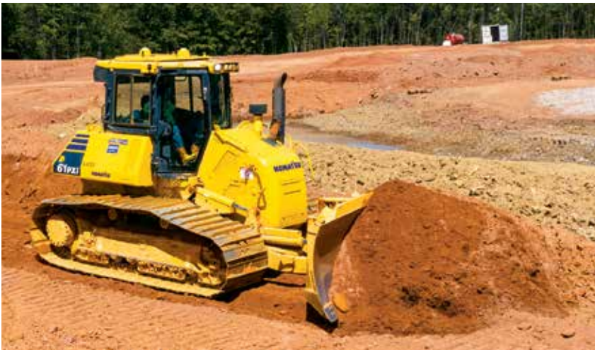
A Komatsu D61PXi-24 IMC dozer gives Triad SC's operators the power and precision to go from rough to fine grading and move material efficiently on large site development projects.
