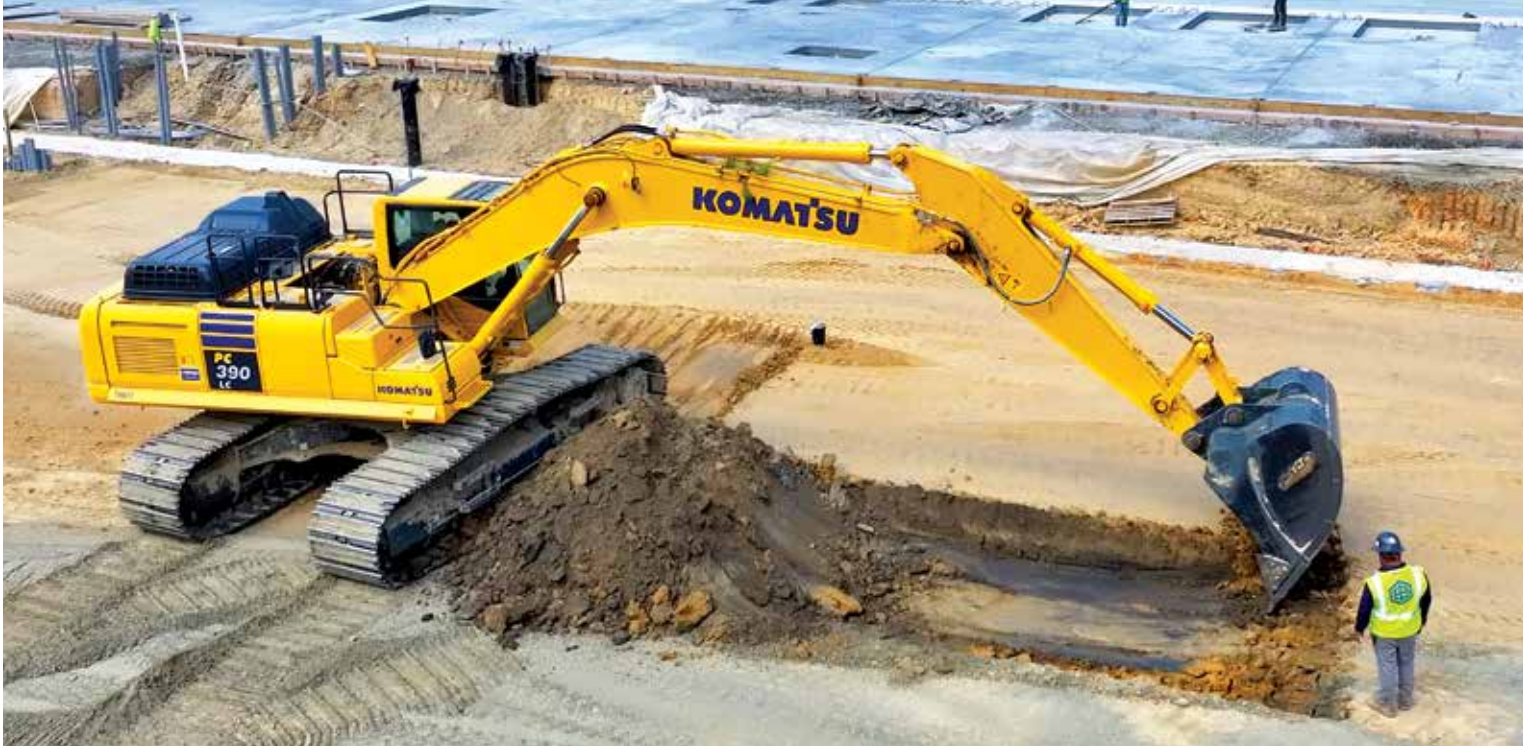
An operator picks up material using a Komatsu PC390LC excavator.
