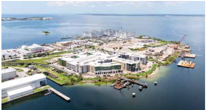
Sitecrafters of Florida Inc. is currently working on a multifamily project.
