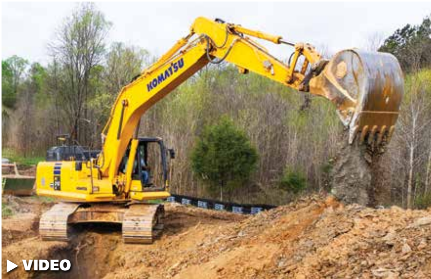
Elite infrastructure Group uses a Komatsu PC210LC excavator to cut a trench for utilities.
