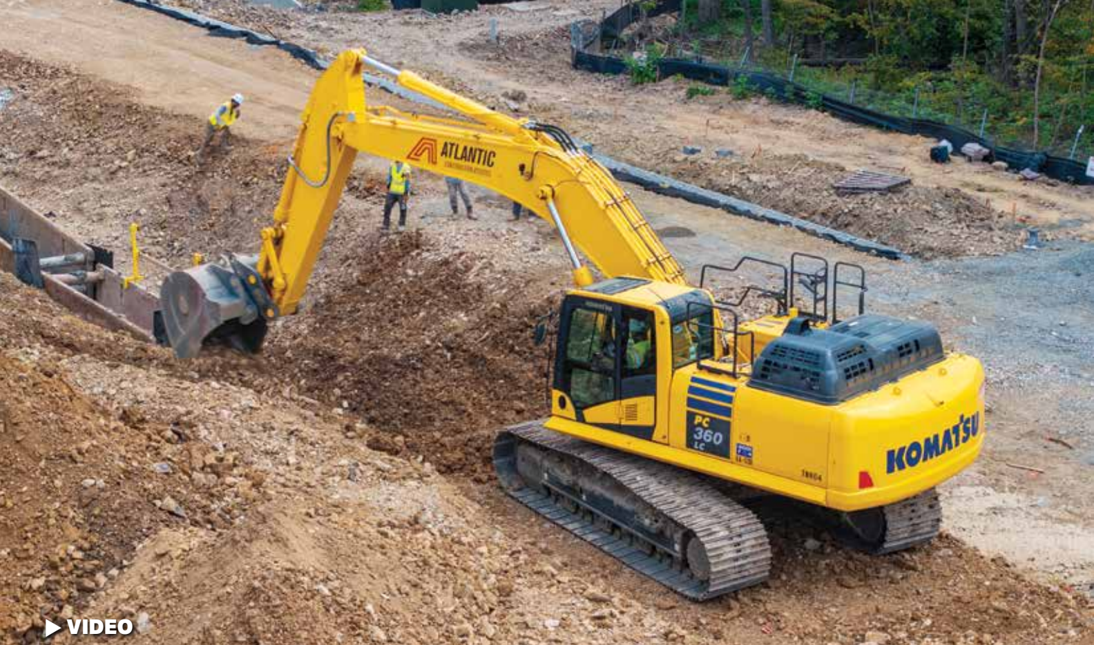
An operator cuts a trench at a data center using a Komatsu PC360LC-11 excavator.
