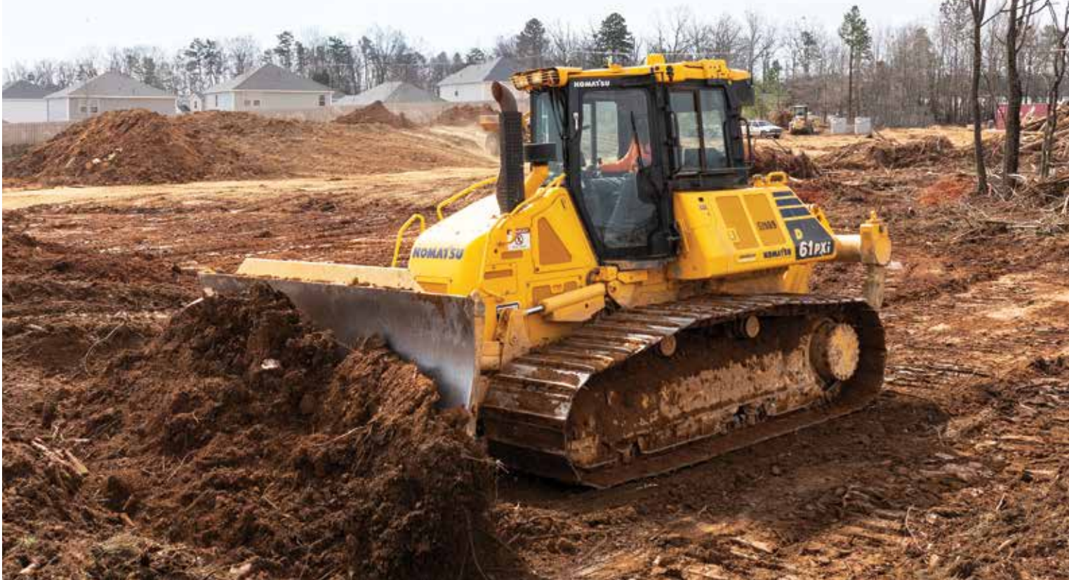
At a Kennedy Excavating jobsite, an operator piles up material with a Komatsu D61PXi-24 IMC dozer.
