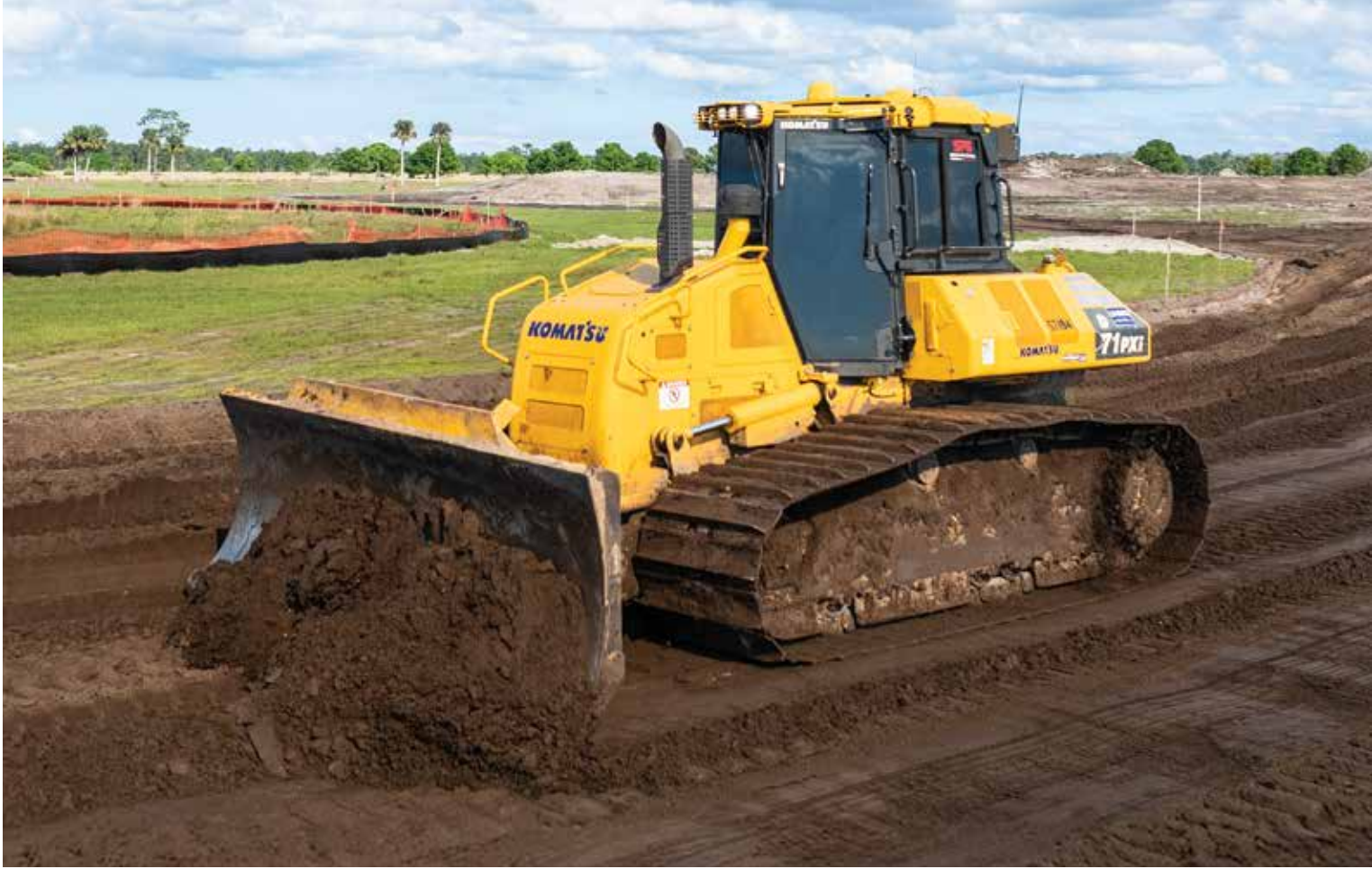
Komatsu IMC equipment, like the D71PXi-24 dozer, help South Florida Grading complete projects efficiently.
