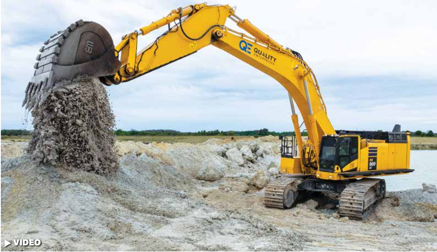
► VIDEO QE primarily uses its Komatsu PC900LC-11 excavator for heavy excavation following blasting operations.
