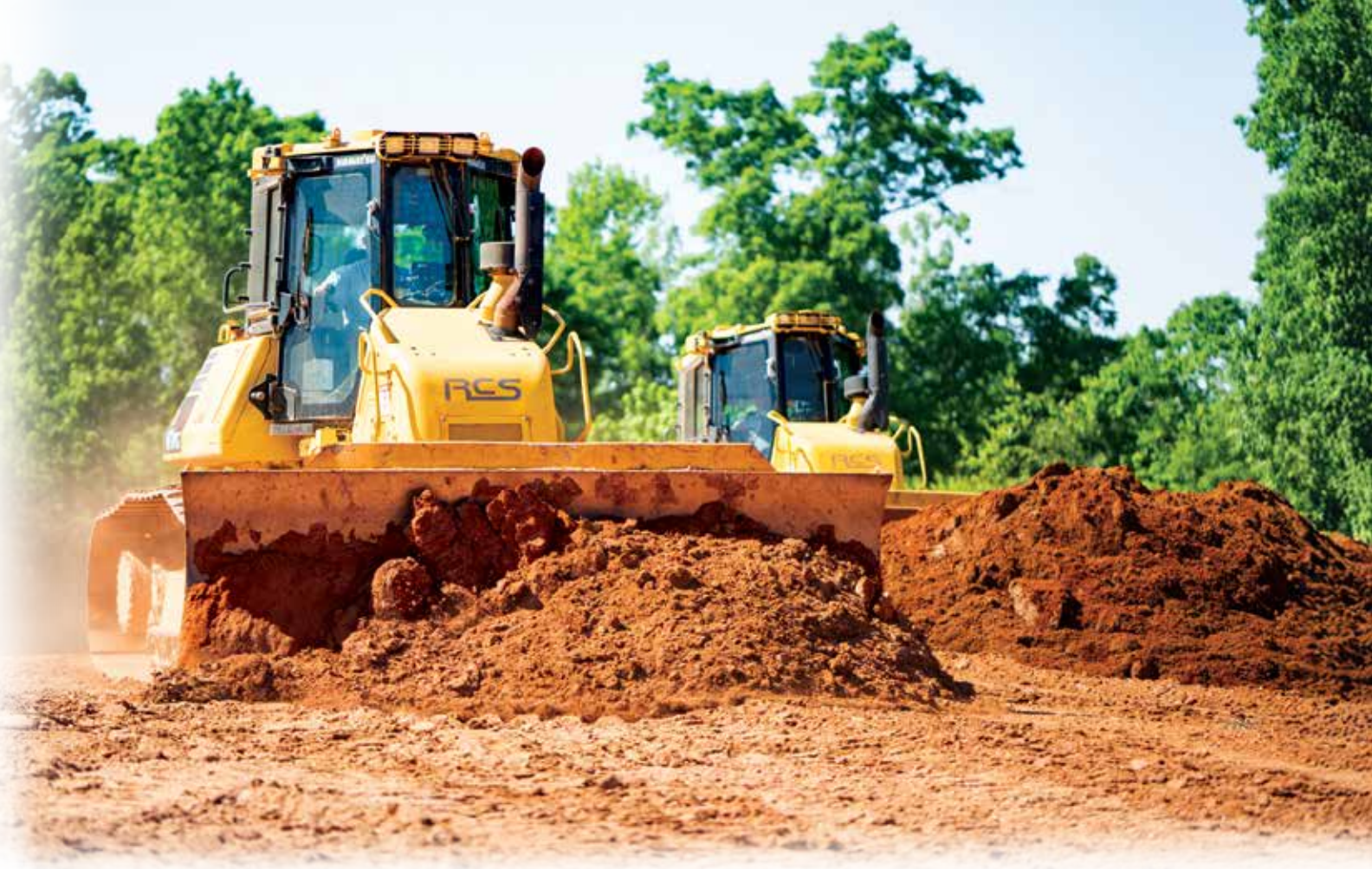
A pair of operators grade a site with Komatsu Intelligent Machine Control (IMC) dozers.
