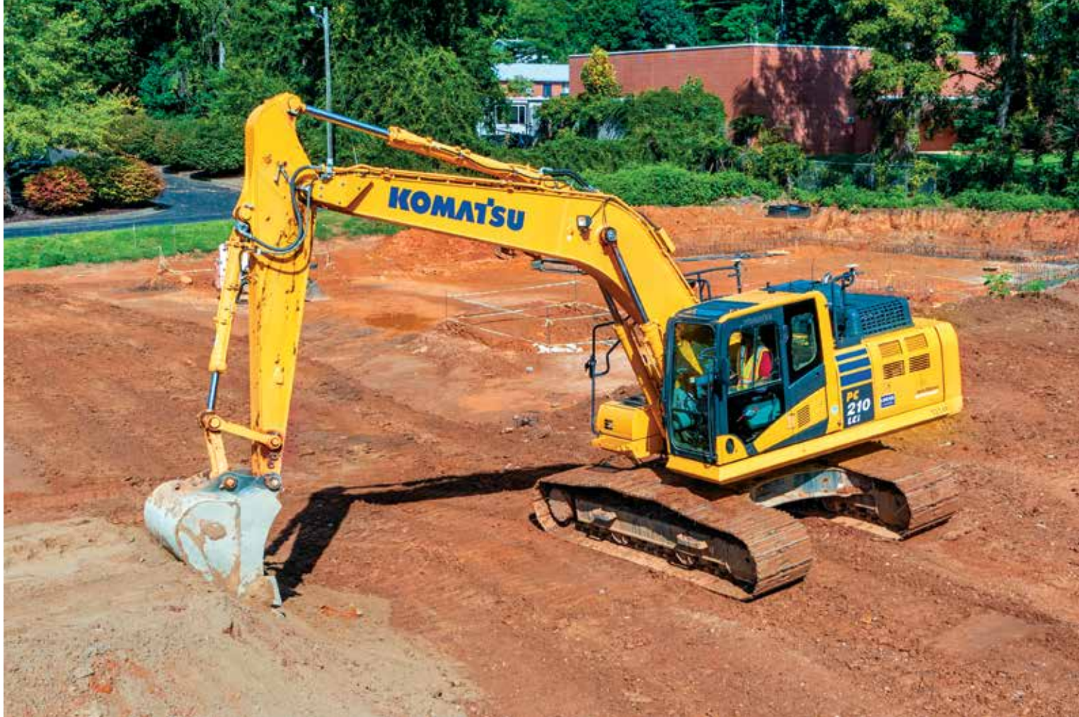
At Patton Construction's apartment complex job site, an operator undercuts a bench with a Komatsu PC210LCi-11 iMC excavator. "The machine allows us to control costs when we're digging ditches and adding stone," said Vice President Austin Patton. "If our estimate says that the bottom of the ditch needs 6 inches of stone backfill that totals 400 tons, the 210 iMC excavator allows us to hit that number exactly."
