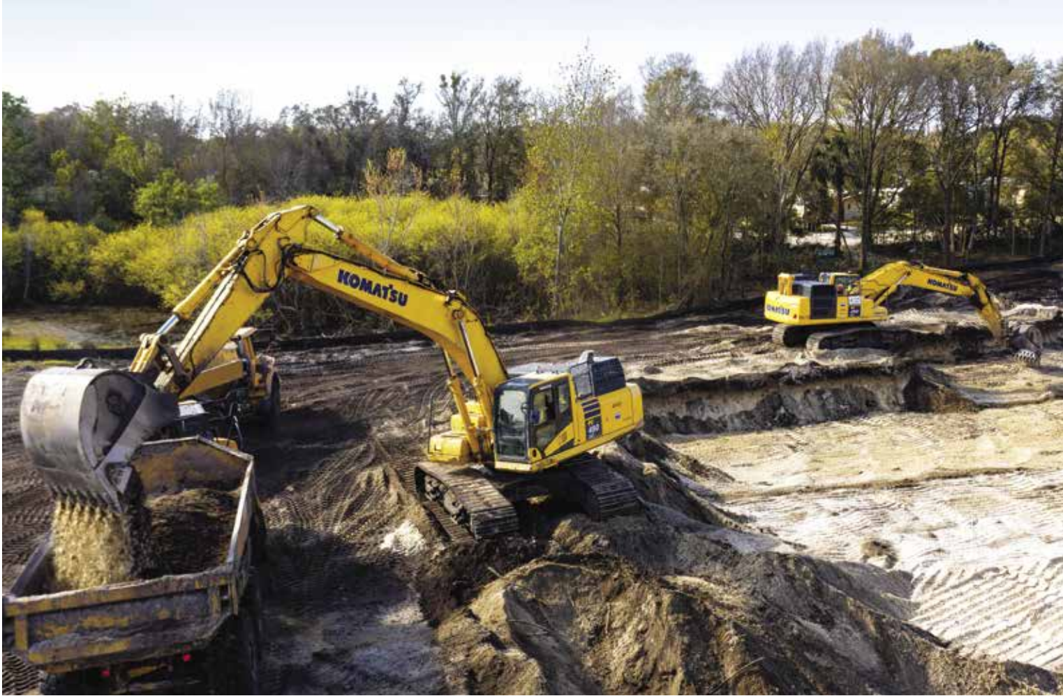
Operators load haul trucks using a pair of Komatsu PC490LCi-11 excavators at a residential subdivision project in central Florida. The excavators use Komatsu's intelligent Machine Control (iMC) with integrated GPS to cut to grade without over digging. "A new operator can receive training in a fraction of the time it used to take and start cutting to grade like somebody that has been operating their whole life," said Chip Tucker, President and Owner of Tucker Paving, Inc.
