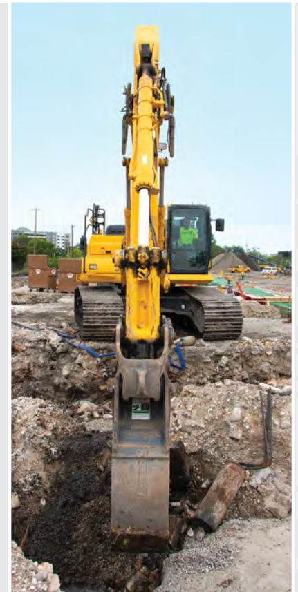
A CornerStone One, LLC operator digs with a Komatsu intelligent Machine Control (iMC) PC360LCi-11 excavator at Komatsu's future global mining headquarters. "With iMC, you can put them right to grade, and once you reach target elevation, it prevents you from overexcavating," said CornerStone One Earthwork Division Manager Scott Christman.
