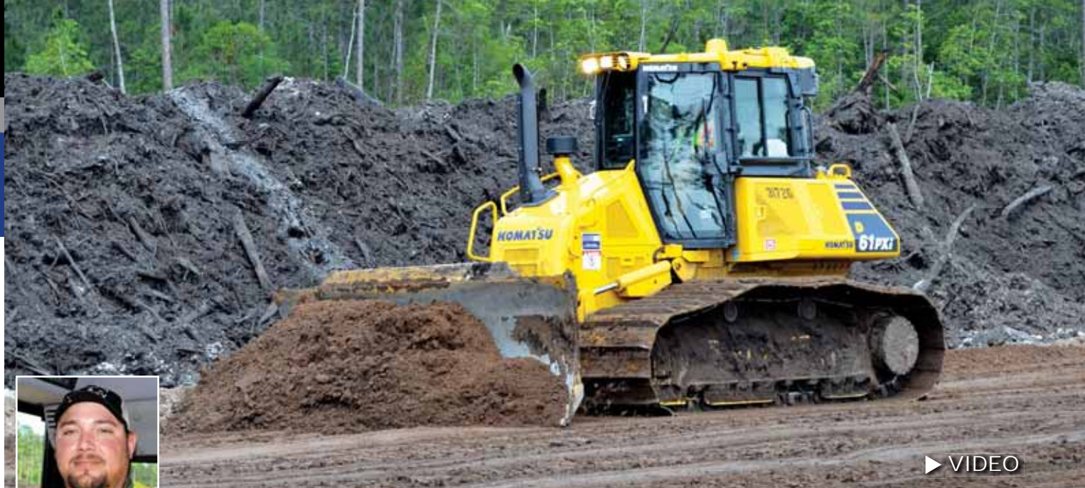
Operator Travis McStephenson uses Capps Land Management's new D61PXi intelligent Machine Control dozer for grading during the State Route 23 reconstruction job in Jacksonville. "The grade-control technology is great," said McStephenson. "The D61PXi is very strong and is also a nice finish dozer."
