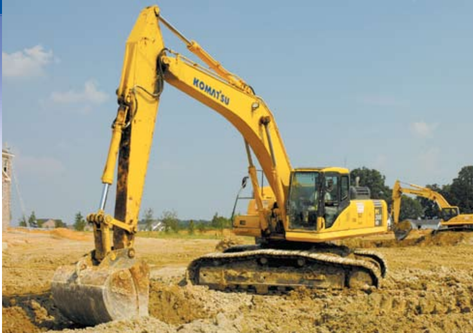
Hoopaugh operators use the company's two Komatsu PC300HD-7 excavators in tandem to move dirt at the Marvin Creek subdivision project in Marvin, N.C. Hoopaugh Grading moved more than a million yards of dirt on the project and handled the entire site-preparation package, including clearing, utility installation and curb and gutter work.
