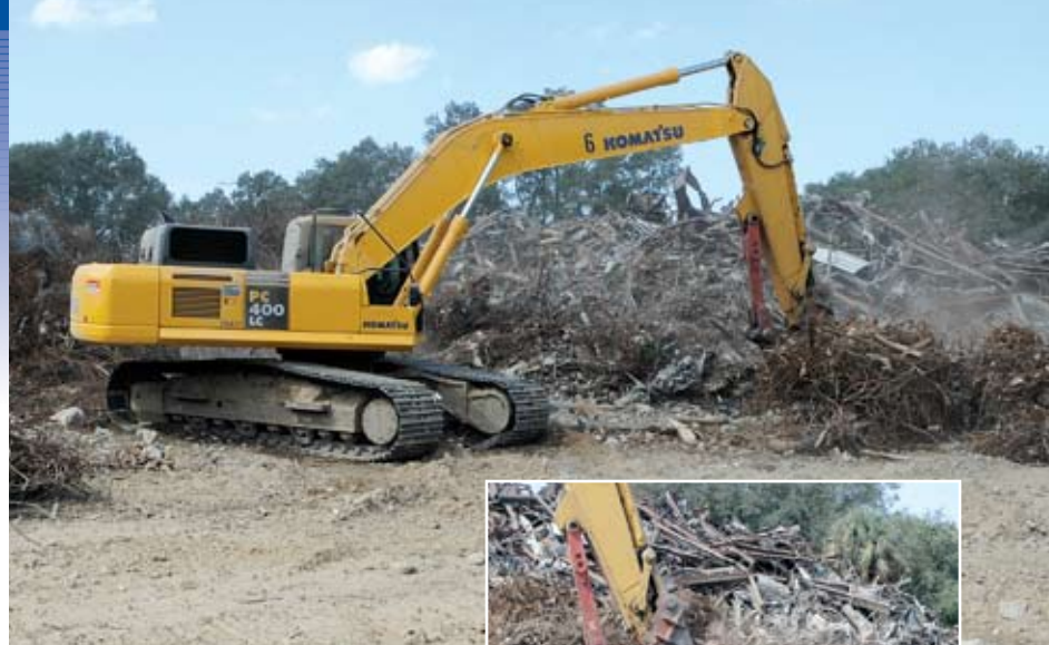
Kuei Tyan has six Komatsu PC400LC-7 hydraulic excavators equipped with specially modified shears, which allow them to efficiently process rebar and cable.
